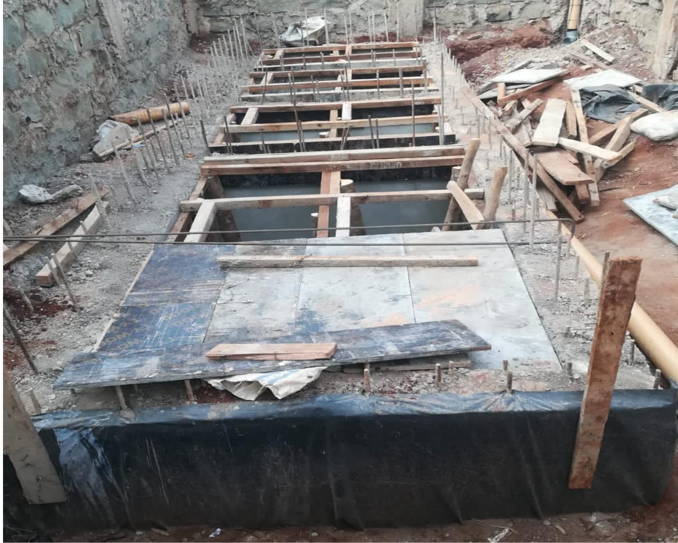
Tank Top Slab formwork & Manholes
